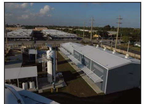
Figure 14. Final Treatment Plant Site with Green Areas, Stormwater Swales, and Improved Site Access (courtesy of CDM Smith)
