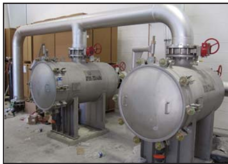
Figure 11. Cartridge Filters Used to Remove Sand and Particulates Prior to Membrane Treatment
