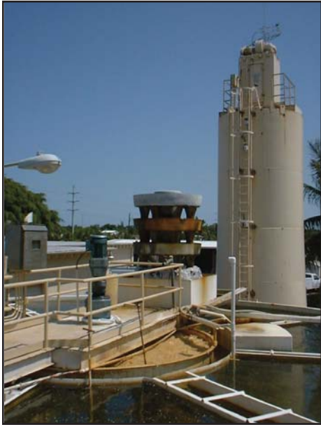
Figure 5. Existing Lime Softening Water Treatment Plant
