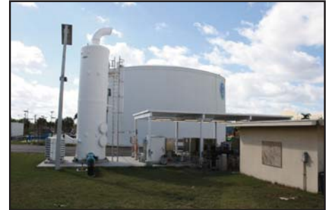
Figure 10. Chemical Feed Systems and Post-Treatment Degasifier to Remove Excess Carbon Dioxide
