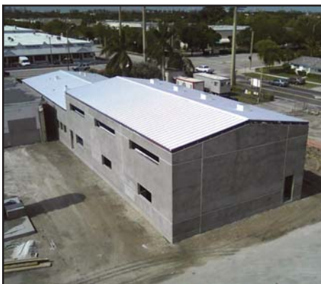
Figure 7. Nanofiltration Building Showing White Reflective Roof (Reduced Heat Island Effect) and Concrete Walls Built From Recycled Local Materials (courtesy of CDM Smith)
