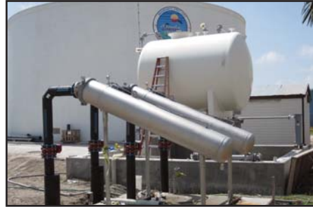
Figure 9. Sand Separators (Local Materials) Used to Remove Bulk of Sand from Raw Water
