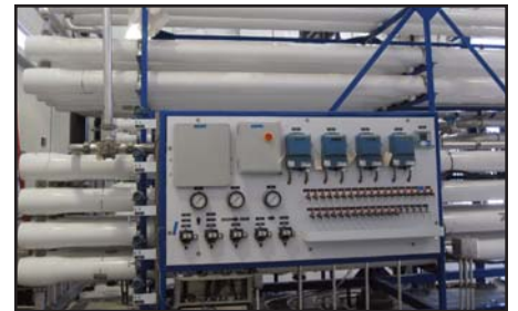
Figure 12. Membrane Skid Testing Bank
