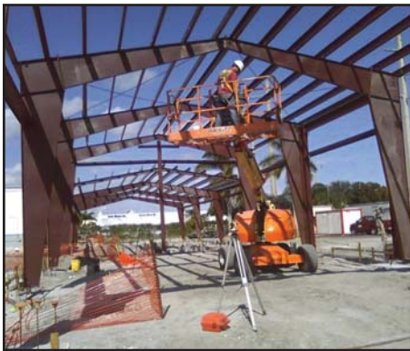
Figure 6. Erection of Steel for Membrane Building Using Recycled Local Materials
